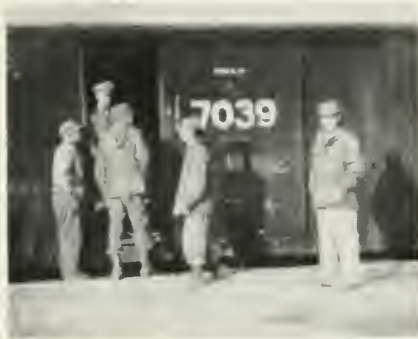
FIELD ENGINEERS BOARD A TROOP TRAIN IN KOREA TO SET UP OPERATIONS AT AN ADVANCED BASE.
